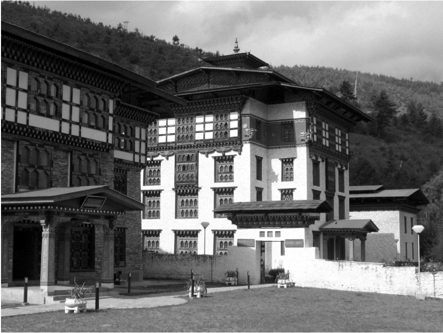
National Library & Archives of Bhutan From left to right: Administration Building, Stack Building housing Choekey Section, Archives Building
