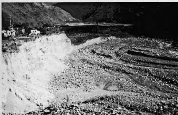
2A. Erosional effects caused by the diversion of the Kali-Gandaki River (1994, April).
