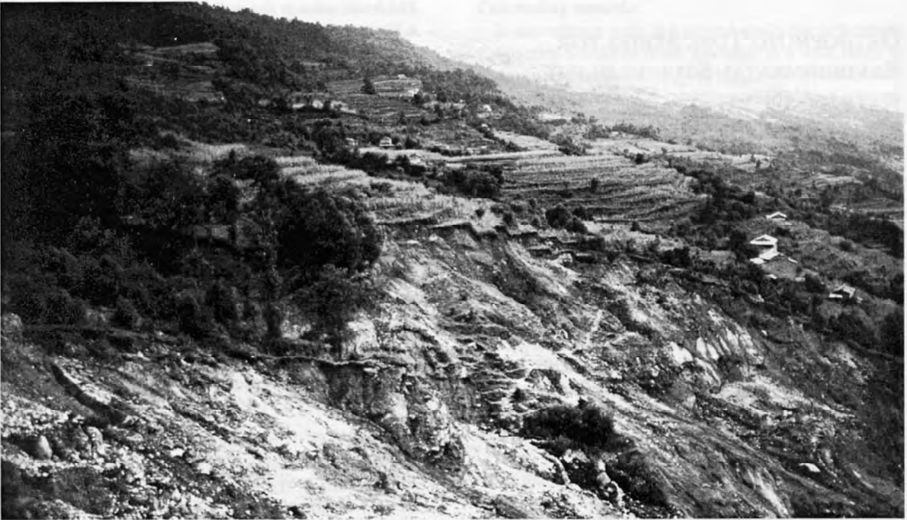
4 A. The landslide of Phalate, east of Sikha (Myagdi District), September 1982.
