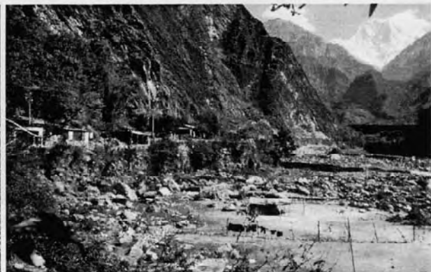
2B. An eroded bank of the Kali-Gandaki River, observed 7 years after the event which created it (1994, April).
