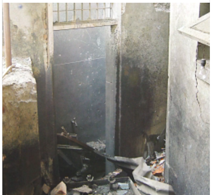
BOMBED: The bathroom of the Triyog Printing Press, adjacent to the Annapurna Post building, caved in after a blast in the early hours Saturday, November 20
