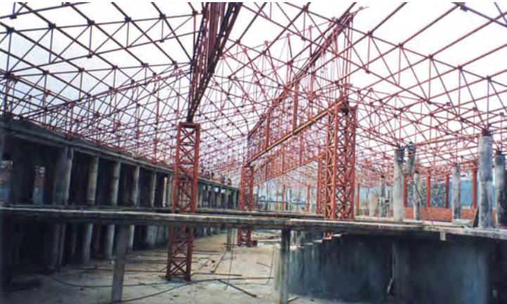
Trusses are going up in the Hall of the Himalaya (above). An architect's rendition of the final building superimposed on an aerial photograph of the site (top).
