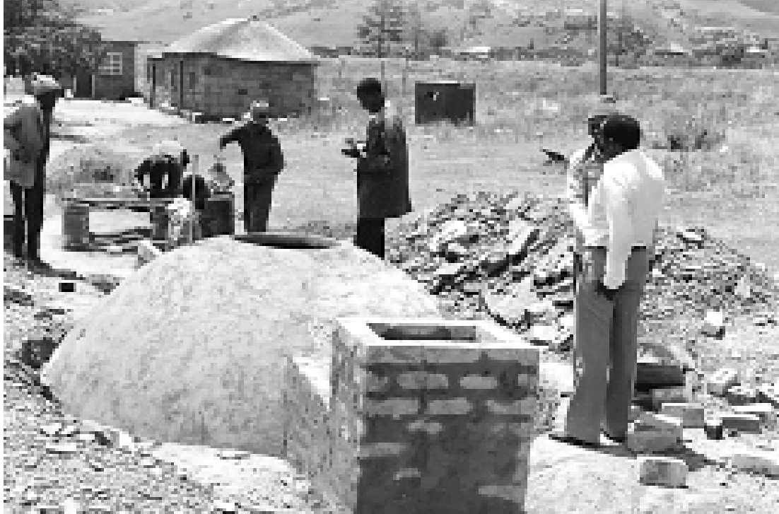
Construction process in building a Nepali design biogas plant in Lesotho.
