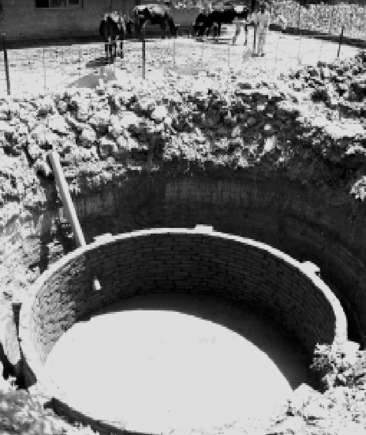
The biogas pit showing the brick lining and intake pipe.
