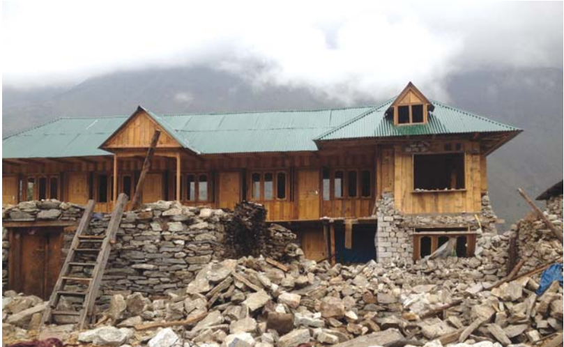
In 2015, the timber frame prevented the complete collapse of a building in Shya La in Nubri even though the outer stone walls fell down (above).
