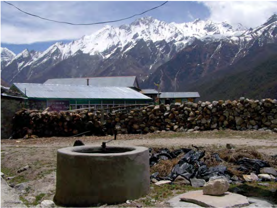
FIRE AND ICE: To make biogas work in cold climates, like this plant in Kyangjin Gompa in Langtang uses a compost heap to insulate the underground digester so the yak dung can be converted into cooking gas.
