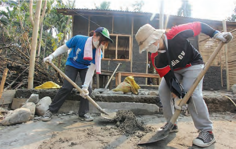
BAMBOO BY BAMBOO: Japanese volunteers help build and renovate old homes in Kakarbhittha, Jhapa, on Sunday, under the Habitat for Humanity initiative of Habitat Nepal.
