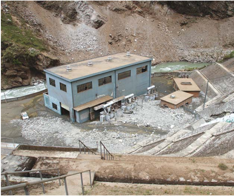
AFTERMATH: The penstock pipe of the Bhoite Kosi hydropower plant ( right ) has been badly damaged, its powerhouse submerged ( left ) and access roads blocked by landslides.
