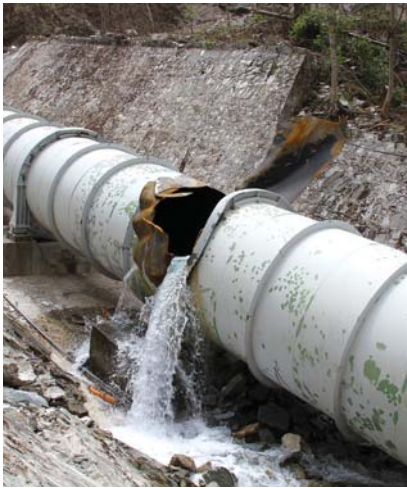
AFTERMATH: The penstock pipe of the Bhoite Kosi hydropower plant ( right ) has been badly damaged, its powerhouse submerged ( left ) and access roads blocked by landslides.
