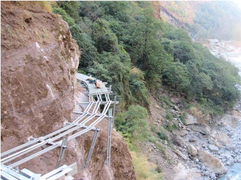
WEEK 6 Fastening steel platforms to cantilever ramps.
