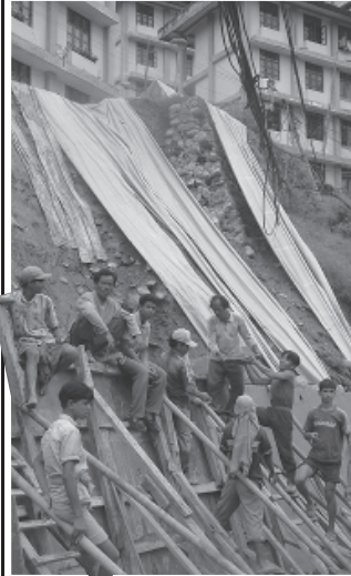
a NOW! pic Work in progress at Syari
