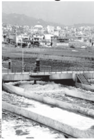
Guliyewari, just north of Pashupati, is set up for sewage separation and water treatment plant, and also 25 hectares of private land along the river to build roads, a 20 metre greenbelt, and embankments. The plant at Kumarigul, Guliyewari, separates sewage entering the river from the Mitra Park and Gokarna areas and filters the water before releasing it into the river beyond Pashupati via an underground tunnel. Sludge, or sediment from the treated water, is pumped into drying beds, and the project hopes to sell or distribute it to the public as fertilizer.
