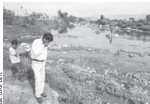
Guliyewari, just north of Pashupati, is set up for sewage separation and water treatment plant, and also 25 hectares of private land along the river to build roads, a 20 metre greenbelt, and embankments. The plant at Kumarigul, Guliyewari, separates sewage entering the river from the Mitra Park and Gokarna areas and filters the water before releasing it into the river beyond Pashupati via an underground tunnel. Sludge, or sediment from the treated water, is pumped into drying beds, and the project hopes to sell or distribute it to the public as fertilizer.
