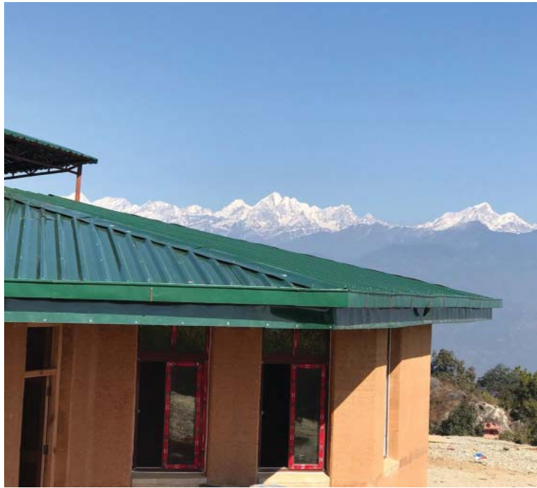
The rammed earth walls insulate the classrooms, make the school ecofriendly, earthquake resistant, and provide protection during monsoon rains.
