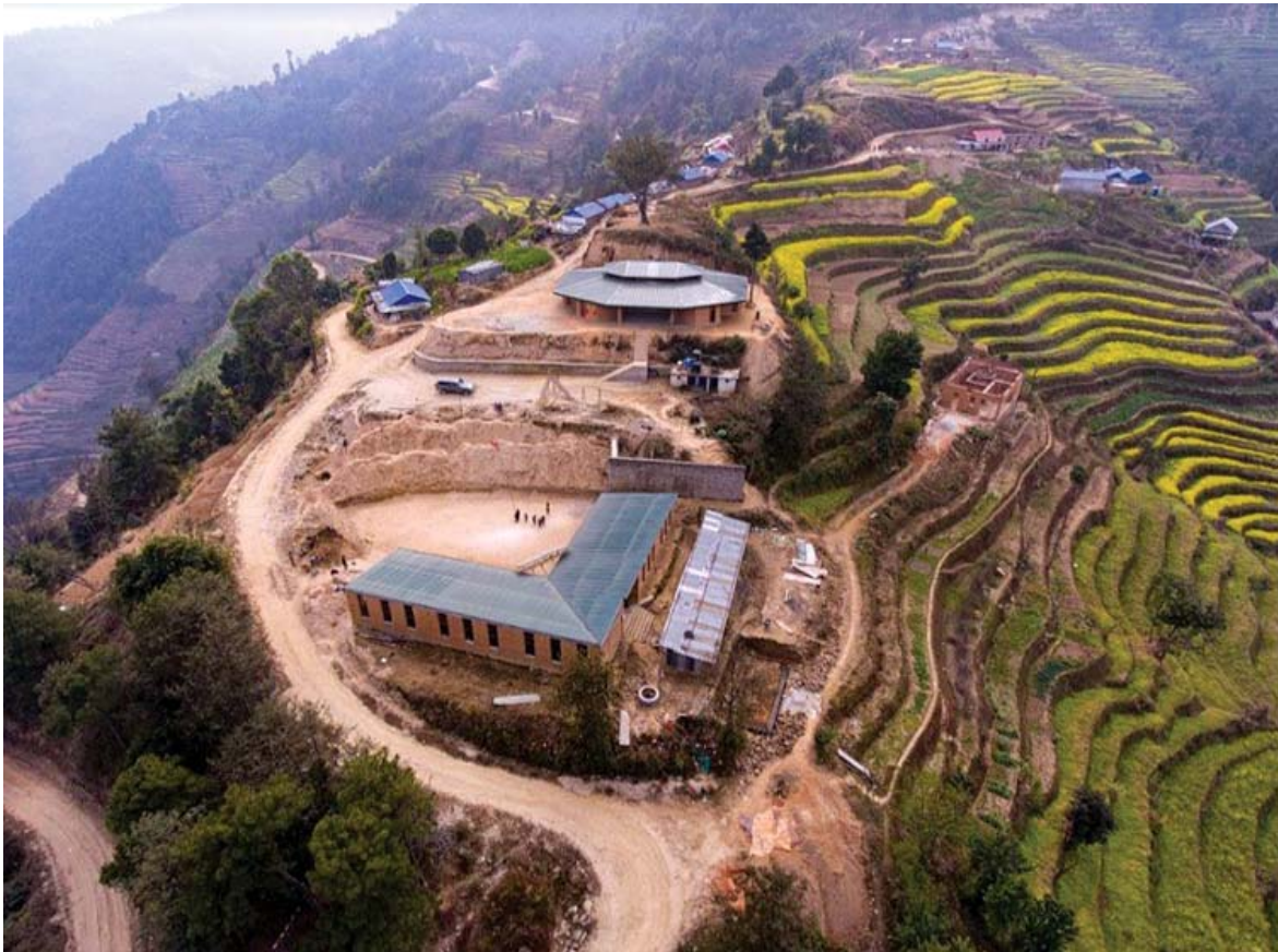
Aerial view of Dwarpaleswor School in Kavre that was completely destroyed in the 2015 earthquake and rebuilt using a seismic resistant rammed earth design.
