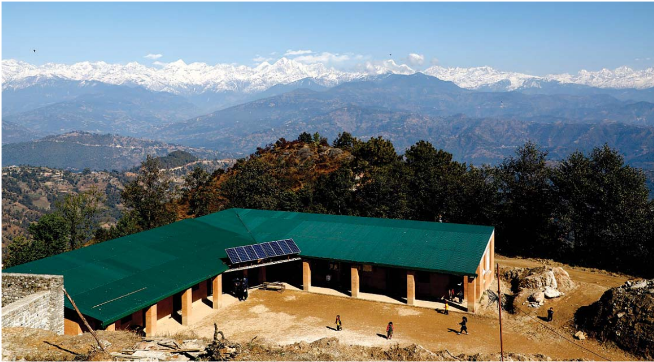
The new building of Dwarpaleswor Secondary School constructed with rammed earth technology hugs the contour of a Kavre mountainside amidst mustard terraces.
