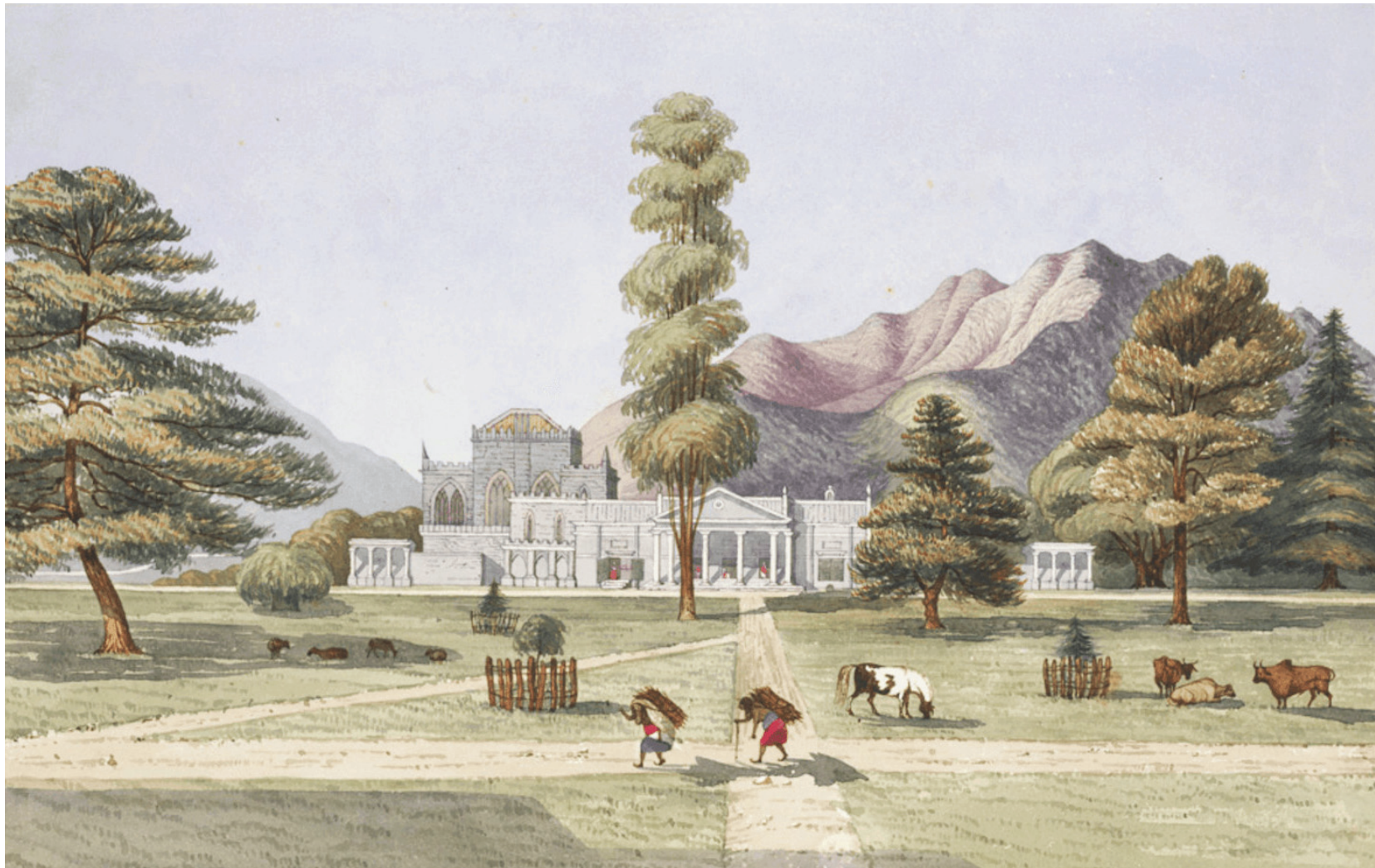
H A Oldfield's 1850 painting of the British Residency in Kathmandu (now the Indian Embassy) showing Nagarjun in the background.
