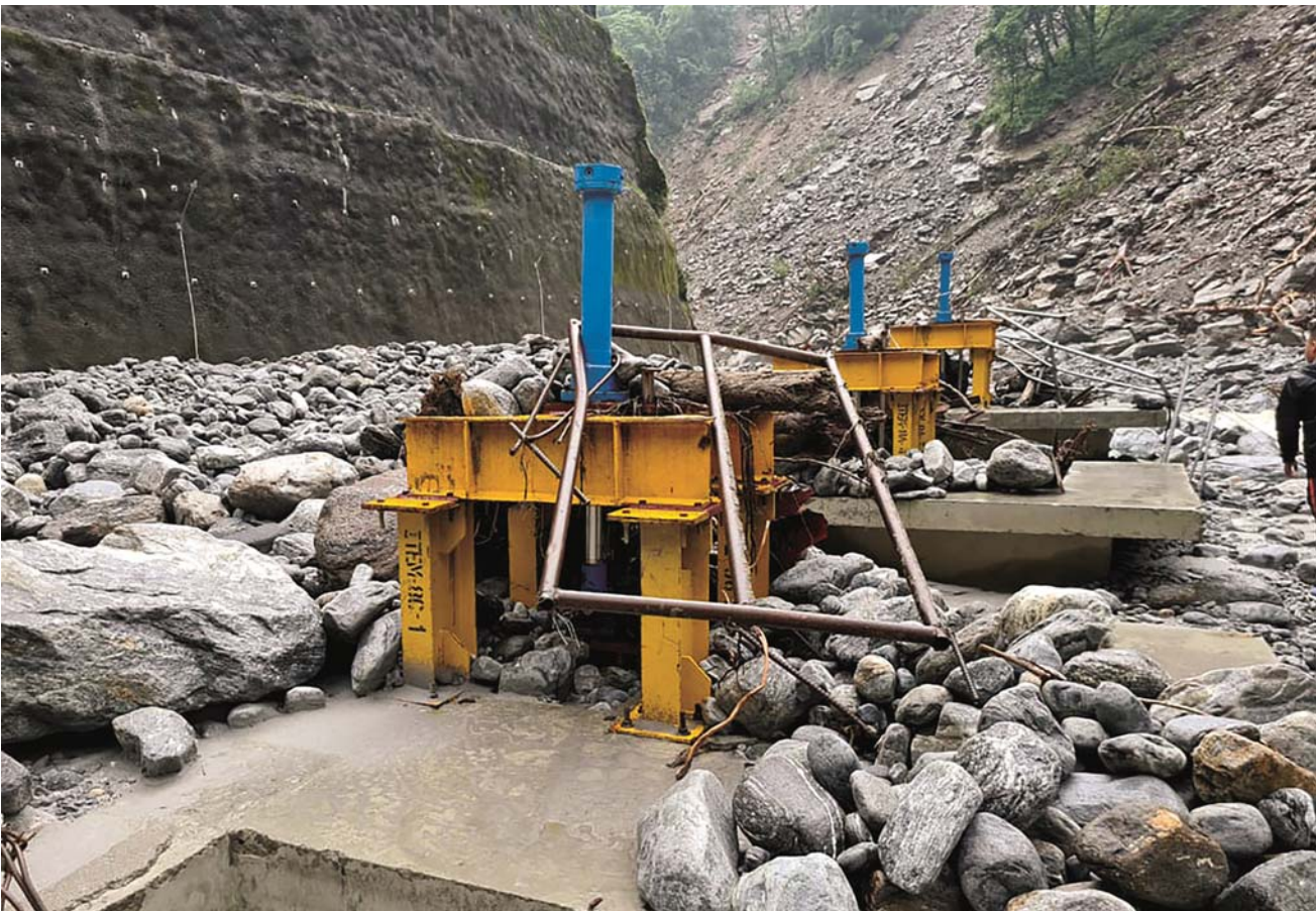
Damage to sluice gates and channel diverting water from the Melamchi to the tunnel at the project headwork. The debris here is 20m deep.
