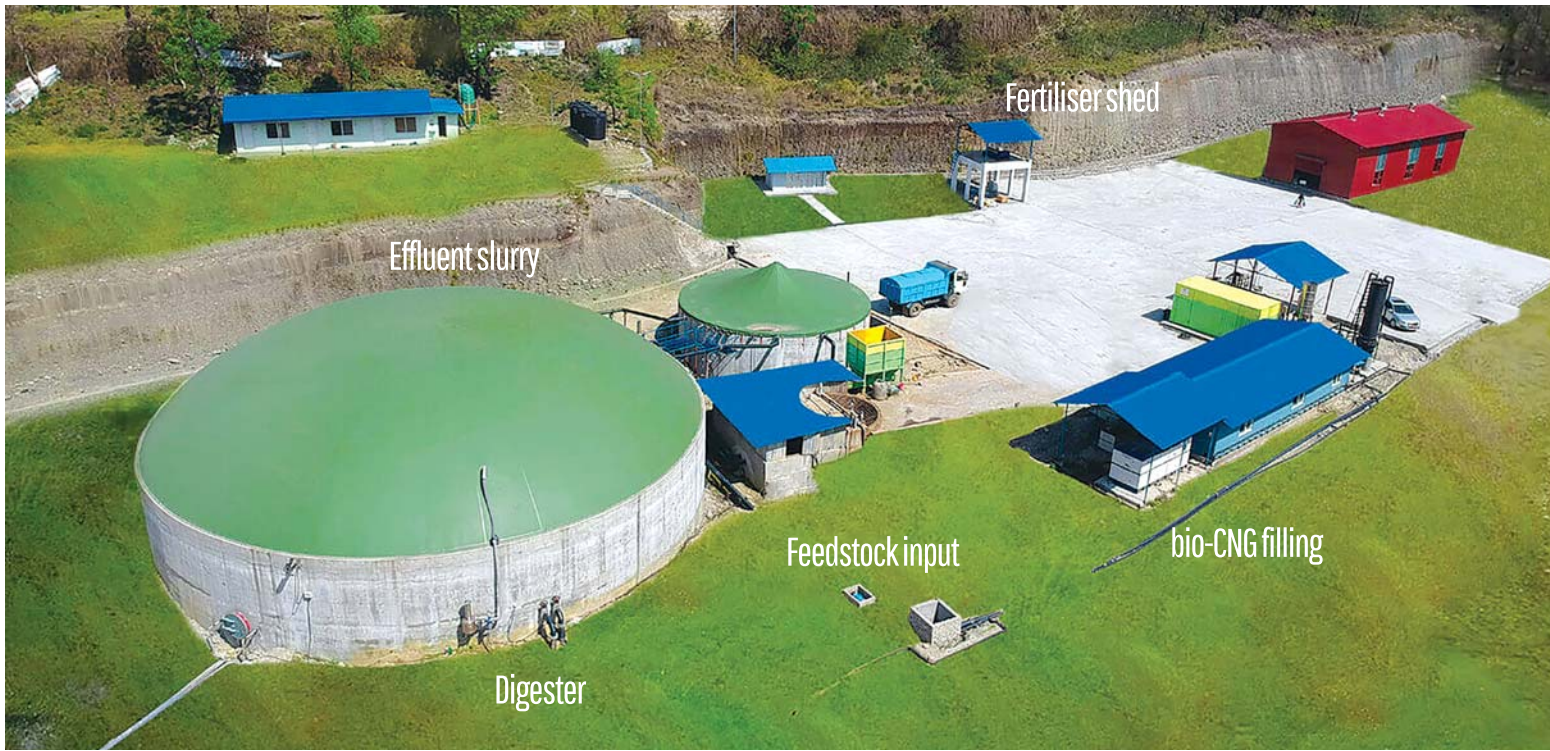
Industrial-scale digester of Gandaki Urja in Kaski.
