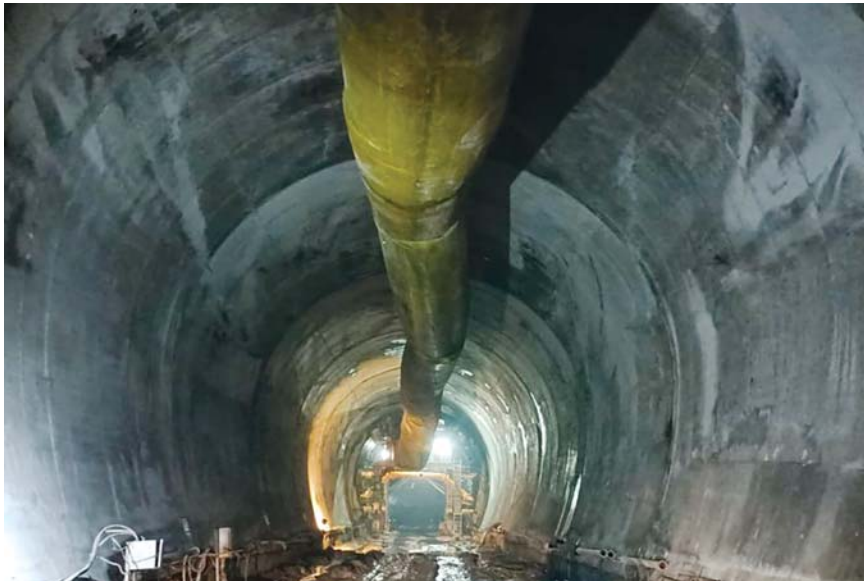
TUNNEL VISION: The headrace tunnel of the 900MW Arun 3 project in eastern Nepal (left).
