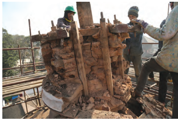
Demolition of the walls revealed hidden structural elements—wooden posts, beams and pegs, that prevented the temple from total collapse.
