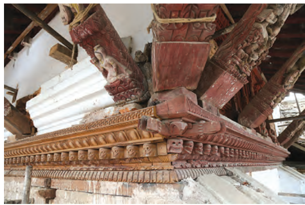
A new five-layered wooden cornice was added to the south facade, duplicating the existing one in the east facade.
