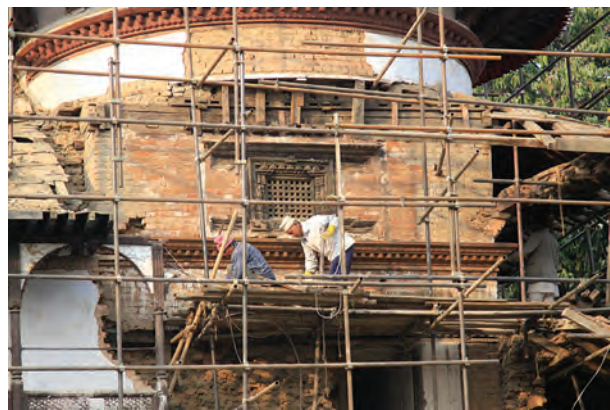
An elaborately carved lattice window had been concealed behind a brick wall during a previous restoration job.
