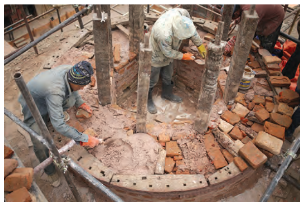
Existing wooden elements and bricks are used without compromising on the added strength and the original ambience of the building.
