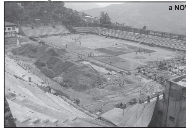
A WORK IN PROGRESS: Paljor Stadium preparing a multi-layered field
